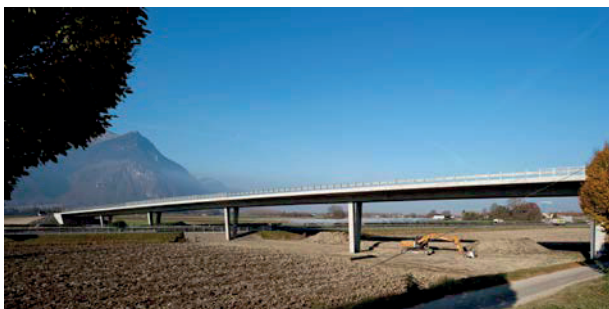
Figure 3: View of the bridge in the straight section
