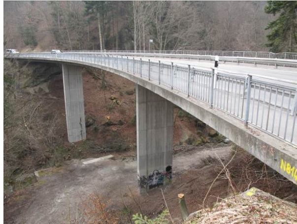
Figure 11: View of the bridge over the Chandelard River
