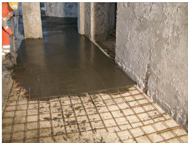
Figure 6: Building in Geneva; preliminary tests of UHPFRC layer
