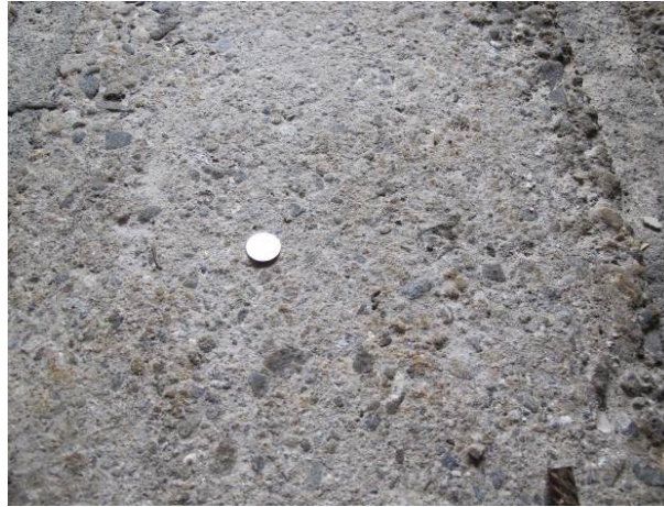
Figure 5: surface of the slab after gritblasting of the building slab in Geneva
