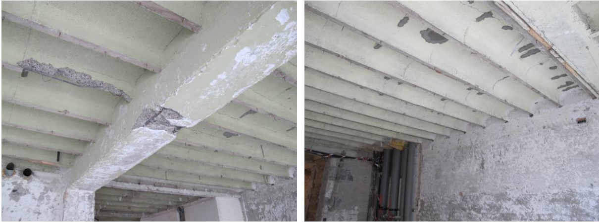
Figure 3: Ribbed slab to be strengthened in Geneva
