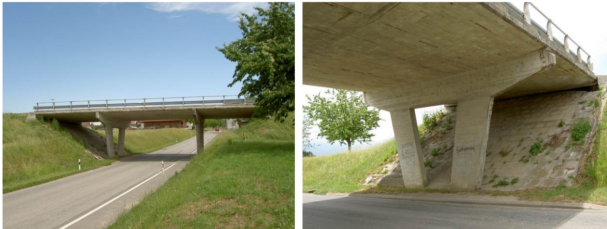
Figure 1: Views of the existing bridge in Vuarrens
