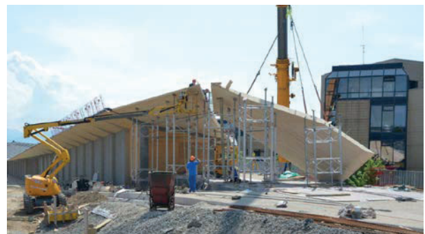
Figure 10: Lifting of the northern roof
