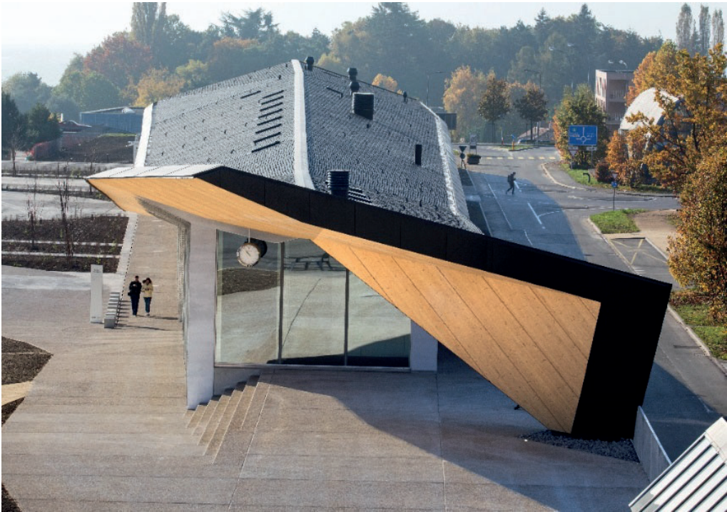
Figure 12: Front view of the northern roof
