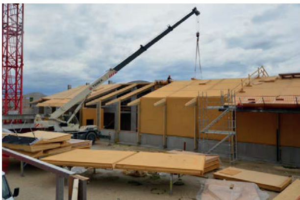
Figure 8: Lifting of the roof
