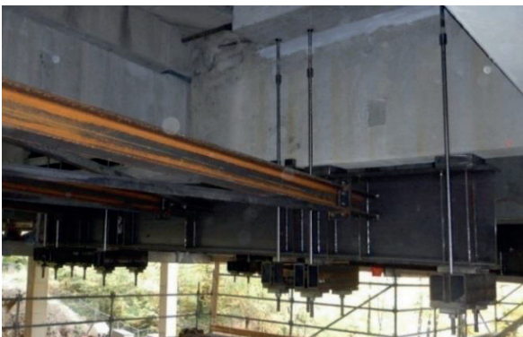
Figure 10. Steel structure supporting the half-joints
