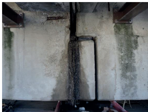
Figure 5. Important water streaming on a half-joint
