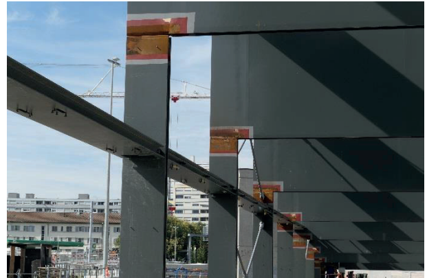
Figure 17. Beam-column on-site welding
