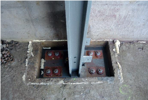
Figure 15. Column footing
