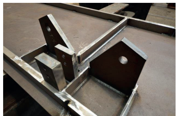
Figure 18. Column-façade beam connections before closing the fourth wall
